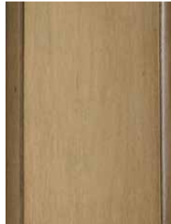
NATURAL Wormholes Filled
